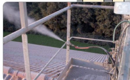
The nebulisation is carried out thanks to simultaneous injections of compressed air and insecticide inside the nozzles specially designed for this process. The formulations are thus dispersed in particulate matter of 5 to 20 microns, according to the air pressure and the throughput required. The nozzles are put in specific places according to the handling methods used.
